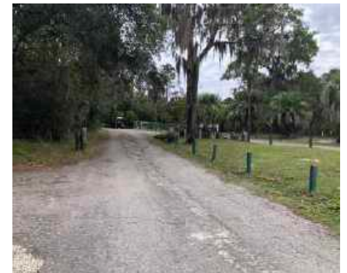
Entry Drive asphalt erosion
